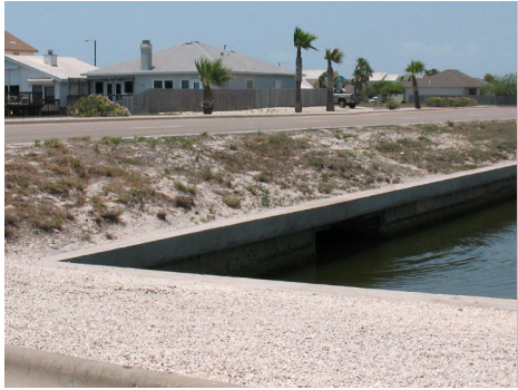
Unimproved canal end
